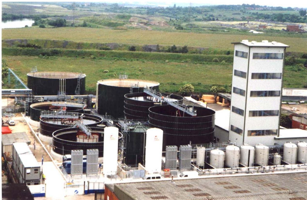
Figure 3: The Vitox ® & Loprox ® facility at Castleford
