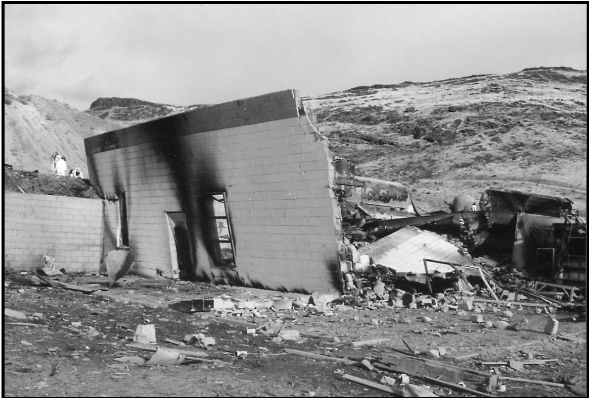
Figure 6. Booster Room 1 After Explosion
