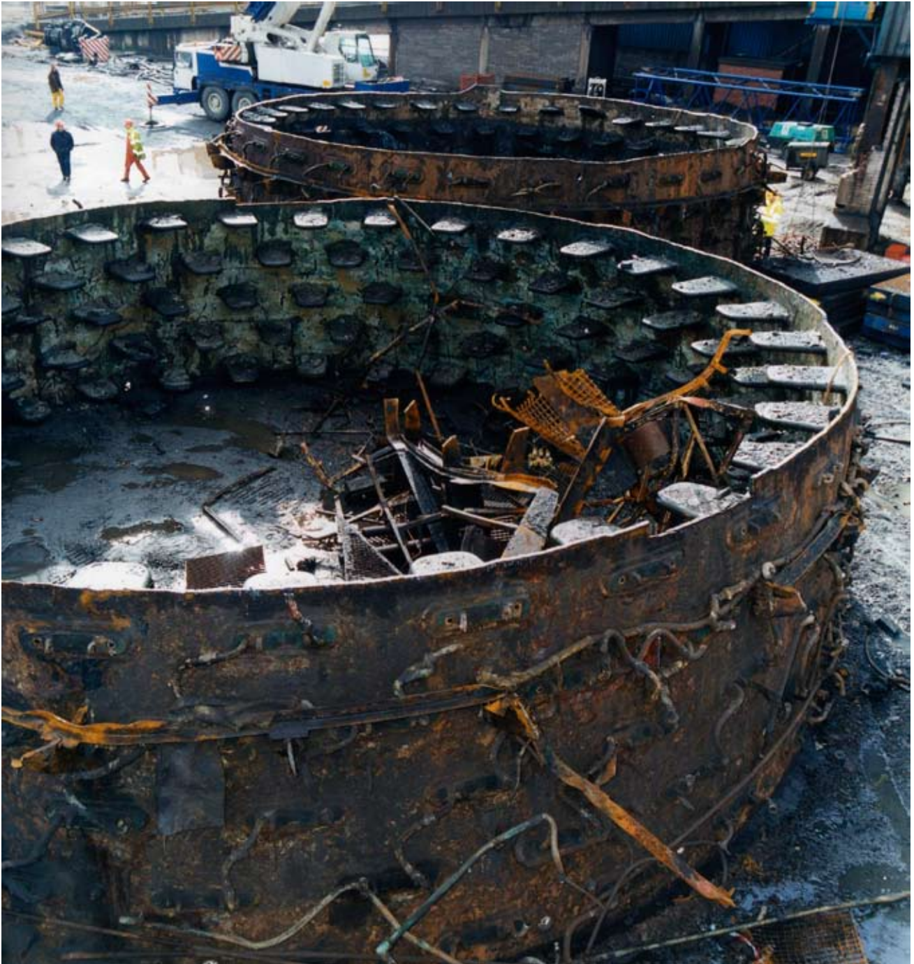
Figure 14 Dismantled furnace section showing coolers
