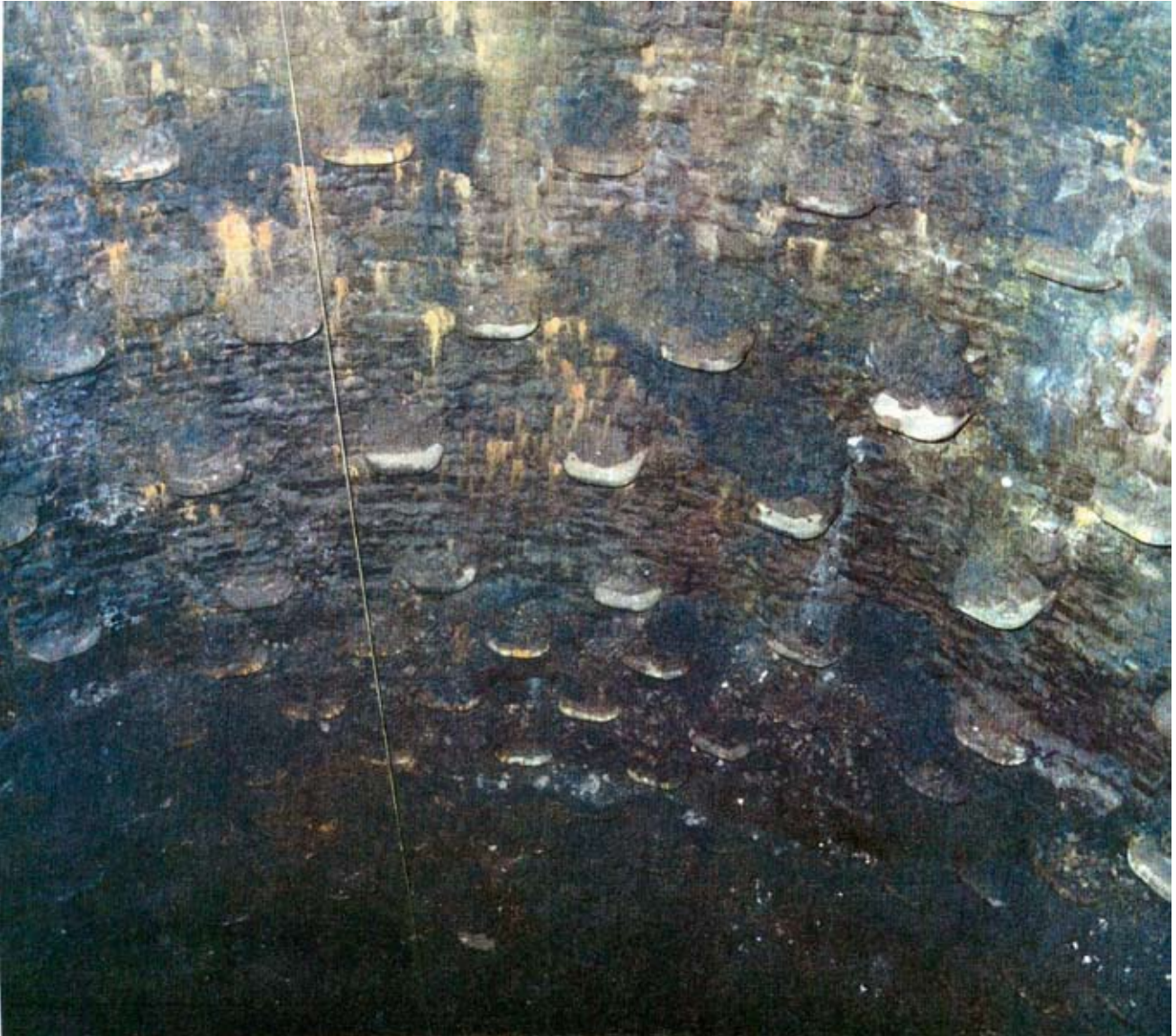
Figure 15 Interior of furnace stack prior to refractory removal
