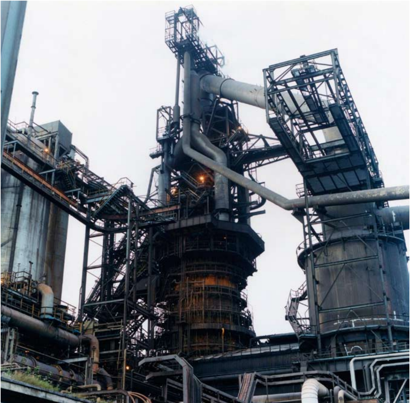
Figure 4 Rear view of No. 5 Blast Furnace
