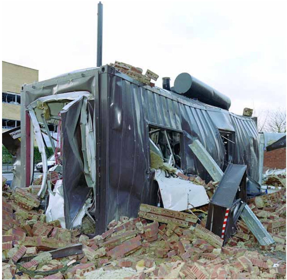
Figure 21 Emergency generator cabin, close to the south-east corner of the Northgate building, viewed from the north east. The north-east segment of the damaged 3-Com building is shown to the left of the picture
