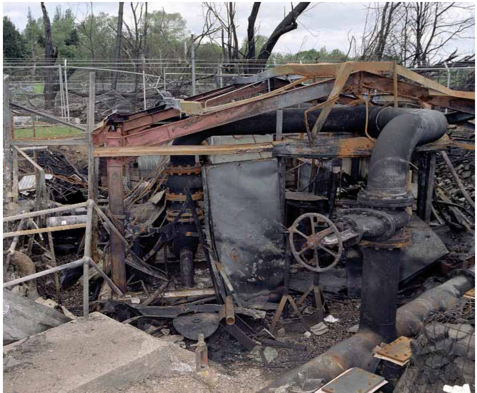
Figure 14 HOSL West emergency pump house from the south-west side. The line of trees behind marks Cherry Tree Lane
