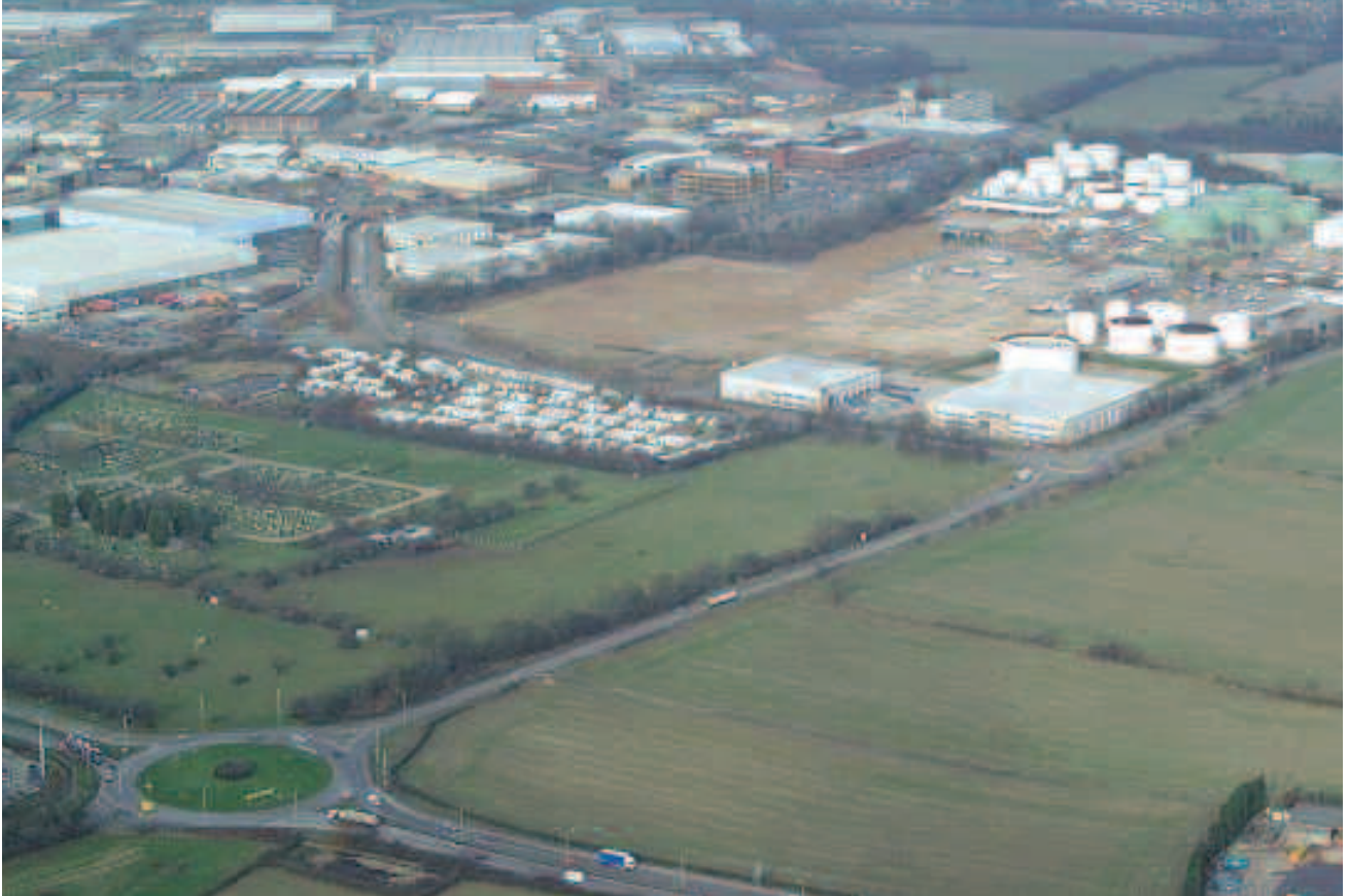
Figure 1 An overview of the Buncefield site and adjacent business and residential communities before the incident
