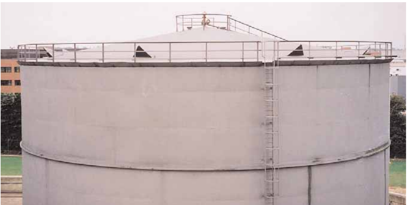
Figure 3 Tank top details before the incident
