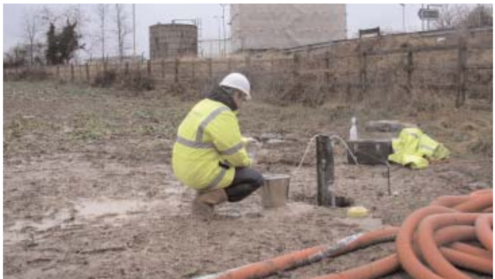
Figure 17 A new borehole at Cherry Tree Lane
