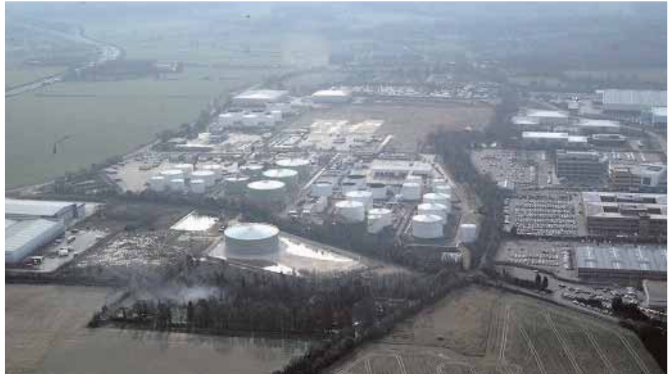
Figure 7 The area prior to incident
