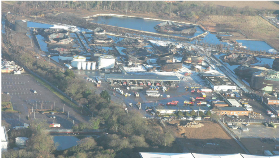
Figure 5 Part of the Buncefield depot after the incident © Chiltern Air Support
