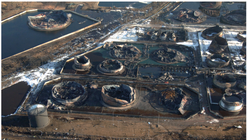
Figure 6 Buncefield after the incident: Tank 912 is in the centre foreground and Tank 12 is in the top left of the picture © Chiltern Air Support
