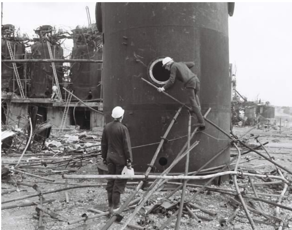
Figure 14: Reverse face of Reactor 5 showing asymmetry in damage.
