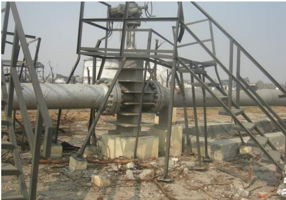
Figure 25: Lightweight open steel structures in the centre of the Jaipur explosion
