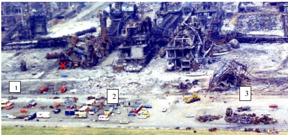
Figure 6: Aerial view of the Flixborough site after the incident – release point marked X
