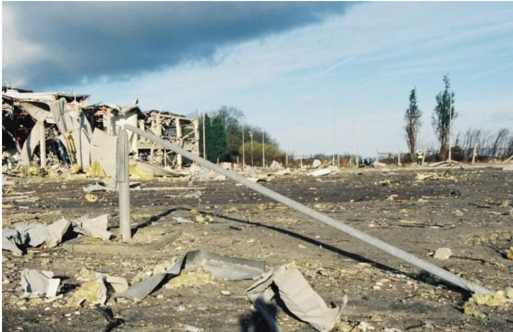
Figure 24: Typical deformation of a lamp post at Buncefield
