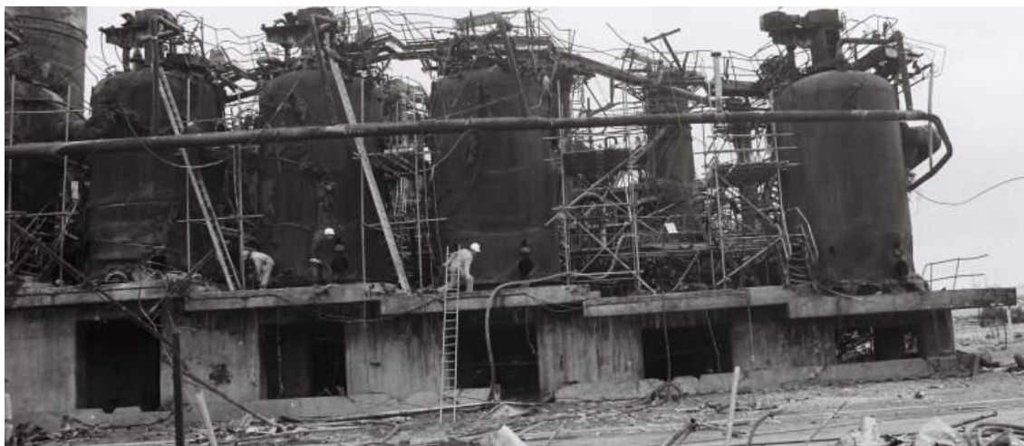
Figure 8: Photograph of part of the reactor train after the incident the dog leg bypass was lost completely. Scaffolding has been erected after the incident.
