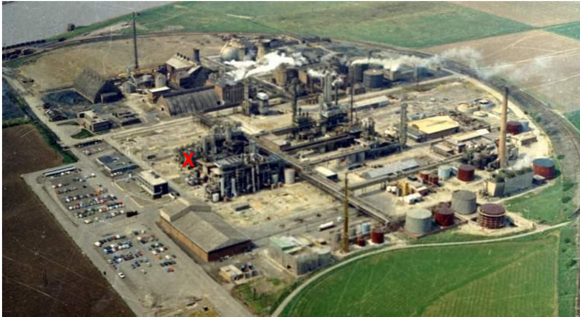
Figure 4: Flixborough site prior to the incident – release point marked X
