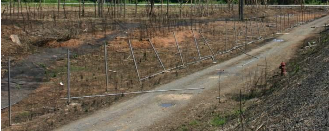
Figure 26: Section of boundary fence in the San Juan incident (CSB, 2015)
