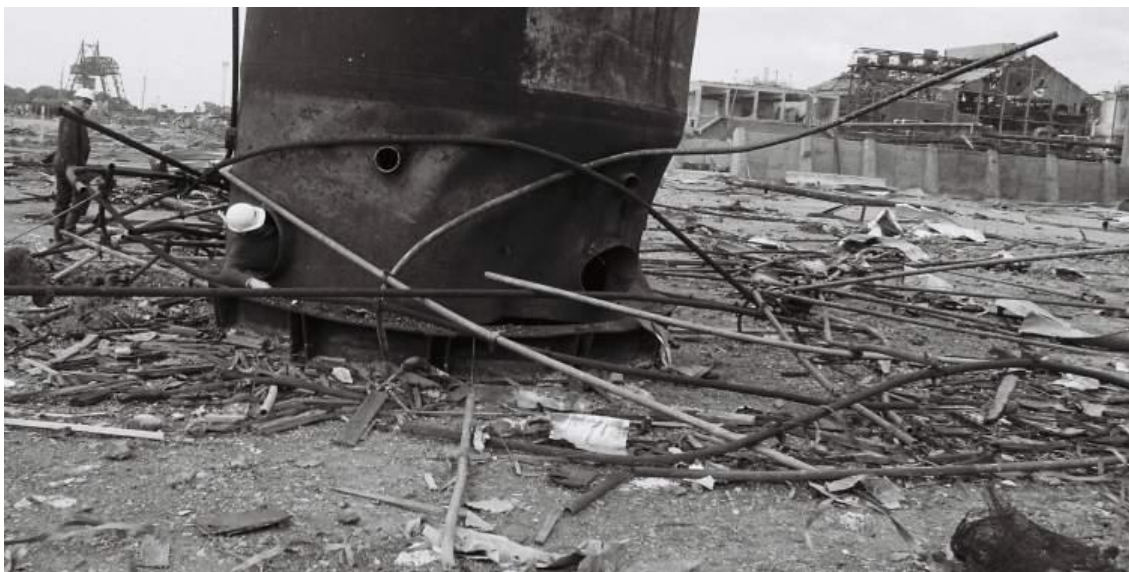
Figure 13: Reactor 5 - Located in open ground approximately 40 m (131 ft) from the leak. Substantial damage to the reactor skirt on the side facing the plant
