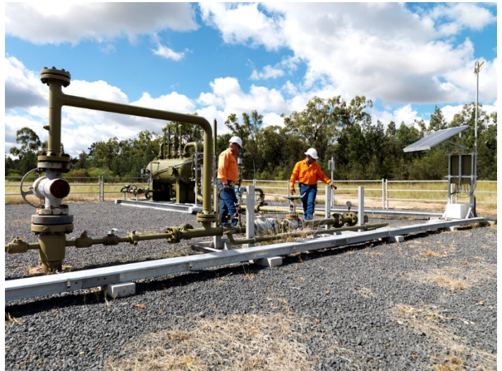
Figure 3: ‘Walking the lines’ (image courtesy of Origin Energy)
