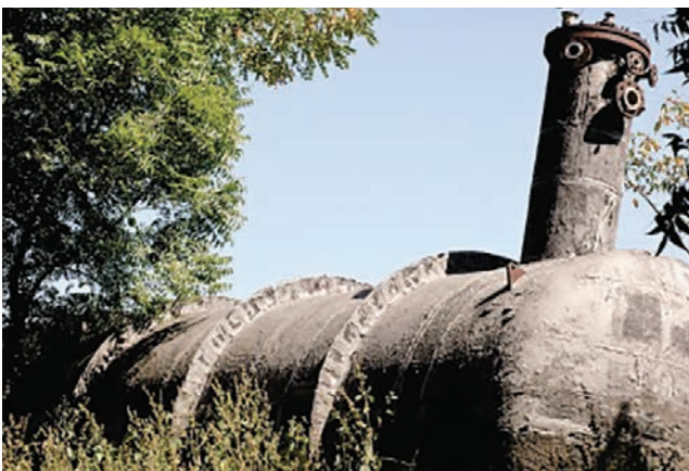
Figure 4: MIC storage tank 610 side-head nozzle configuration.
