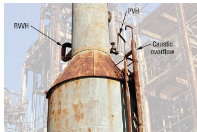
Figure 6: Vent gas scrubber pipe configuration
