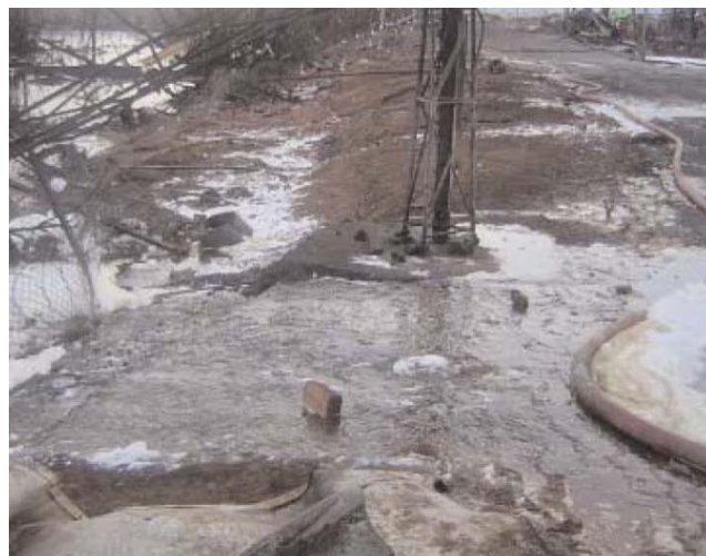
Buncefield: leaking bund wall (top), firewater runoff (bottom)
