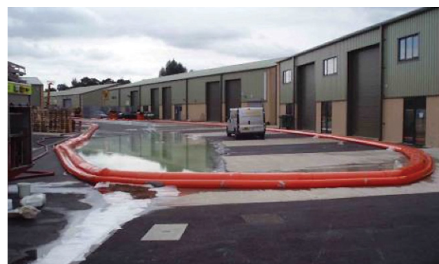
(Top to bottom) Biolab fire: damage and emergency containment
