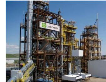
Fuel: MSW. Steam-Oxy gasifier. Scale: 100k tonnes/year input, Technology: Enerkem
