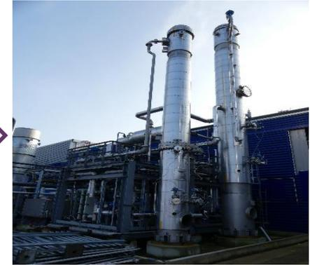
Product separated from by-products ready for sale. Demonstration plant used K<sub>2</sub>CO<sub>3</sub> solution to capture food grade CO<sub>2</sub>. Methane is then injected into grid.
