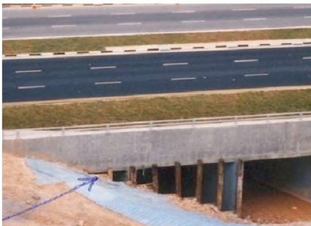
Figure 2a: Restricted access to cell 1 under carriageway
