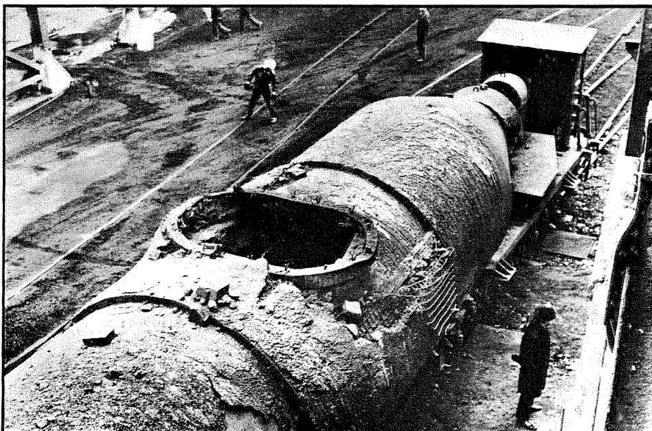
Fig 9 The torpedo concerned photographed shortly after the incident. Metal/slag residues can be seen, and damage to the refractory lining in the throat area
