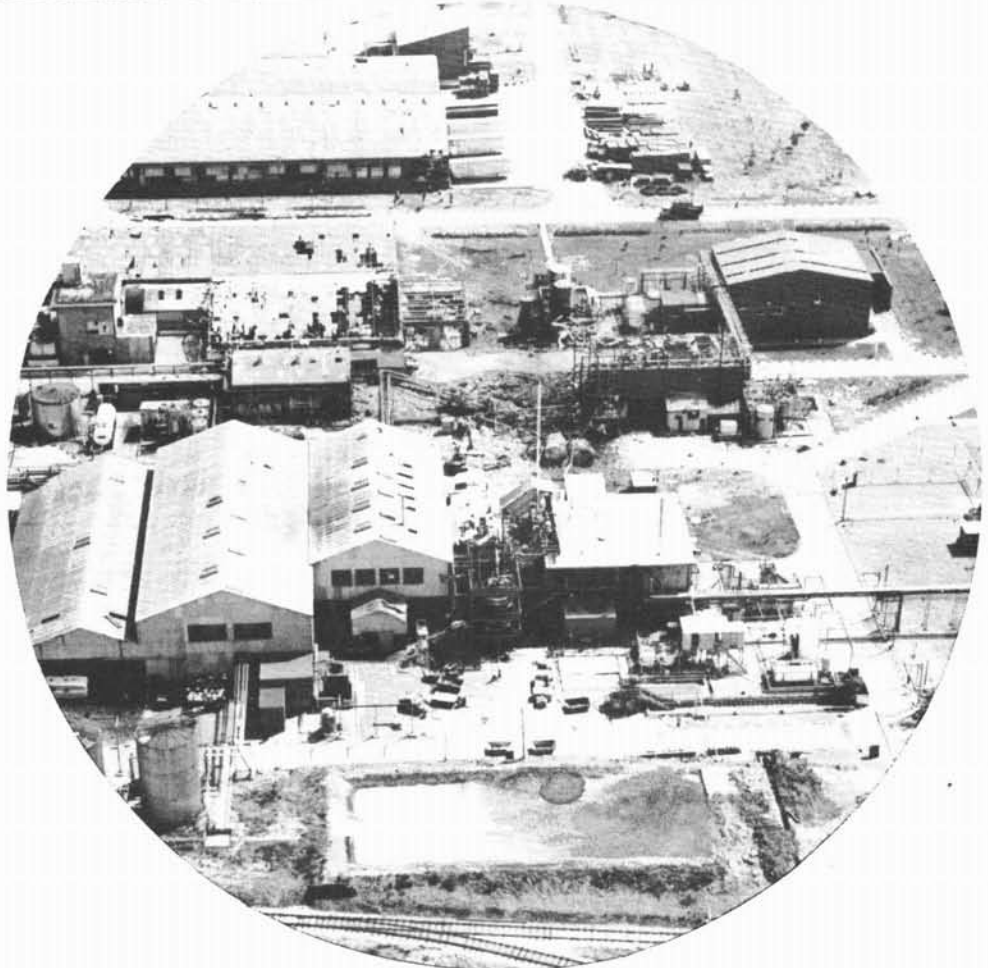
AFTER This photograph is reproduced by courtesy of the Chief Constable of the Norfolk Constabulary. It shows the Clopidol plant at the centre of the explosion (mid-foreground), and damage to the roofs of nearby warehouses. The site plan on the centre pages shows the detail of the plant and the spread of the debris flung out by the force of the explosion.
