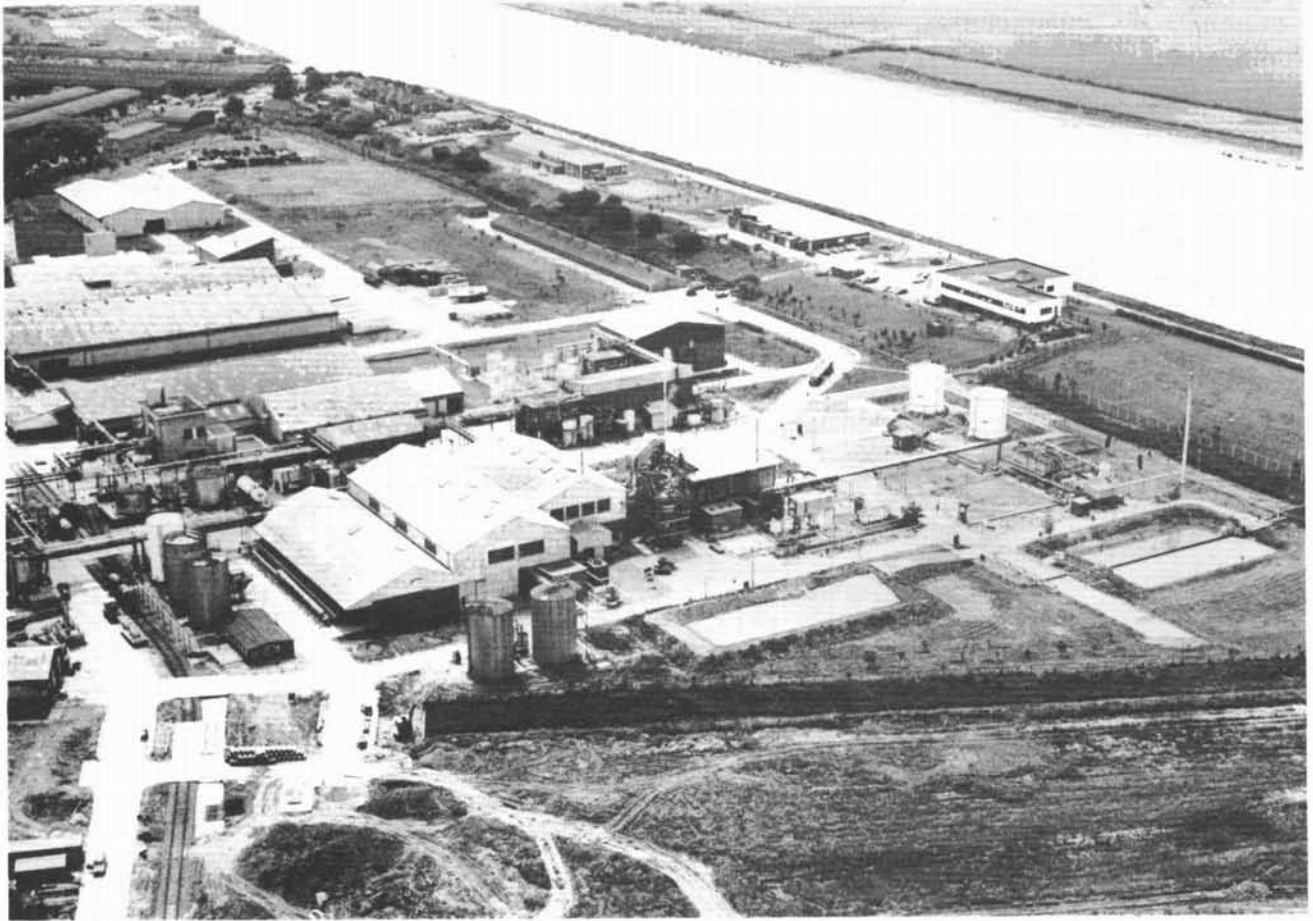
BEFORE An aerial view of the site taken some time before the date of the explosion.
