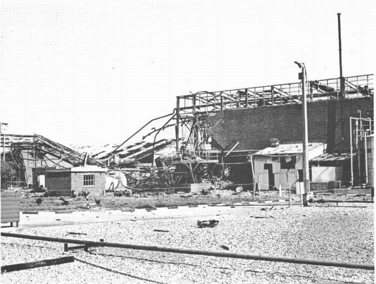
Another view of the Clopidol building showing the collapsed pipe bridge.
