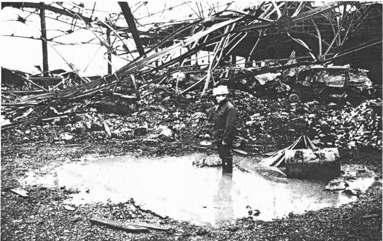
Fig 6 The major crater, No 1 (App 4, Fig 5), with piled remains of milk powder behind.
