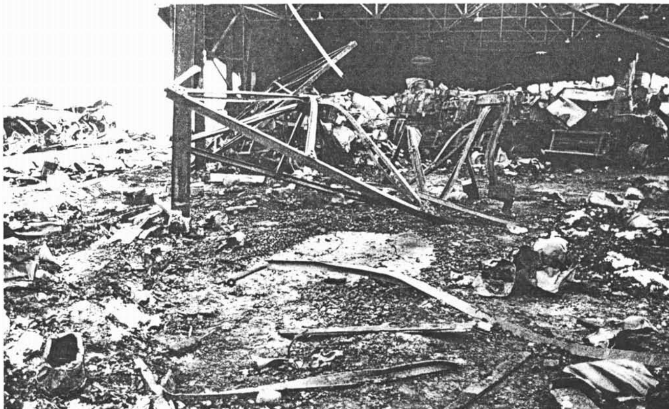
Fig 7 The uprooted stanchion with crater No 5 (App 4, Fig 5) in foreground.
