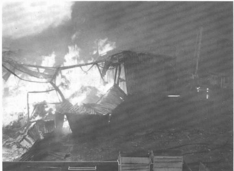
Fire in Unit 1 with collapse of the gable wall South Yorkshire Constabulary
