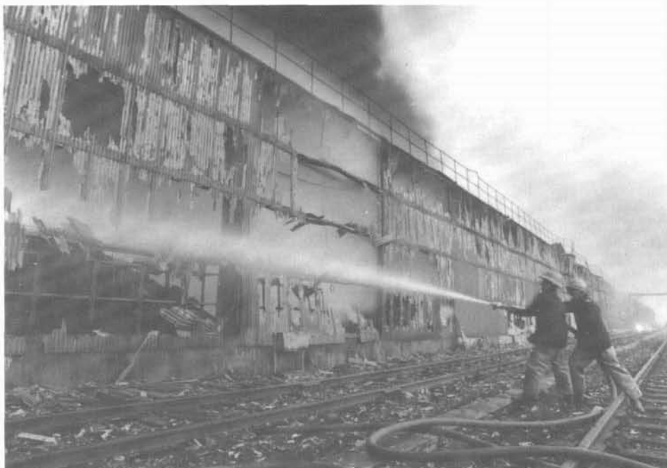
Railway elevation showing exploded asbestos cement sheeting and buckled structure Sheffield City Council
