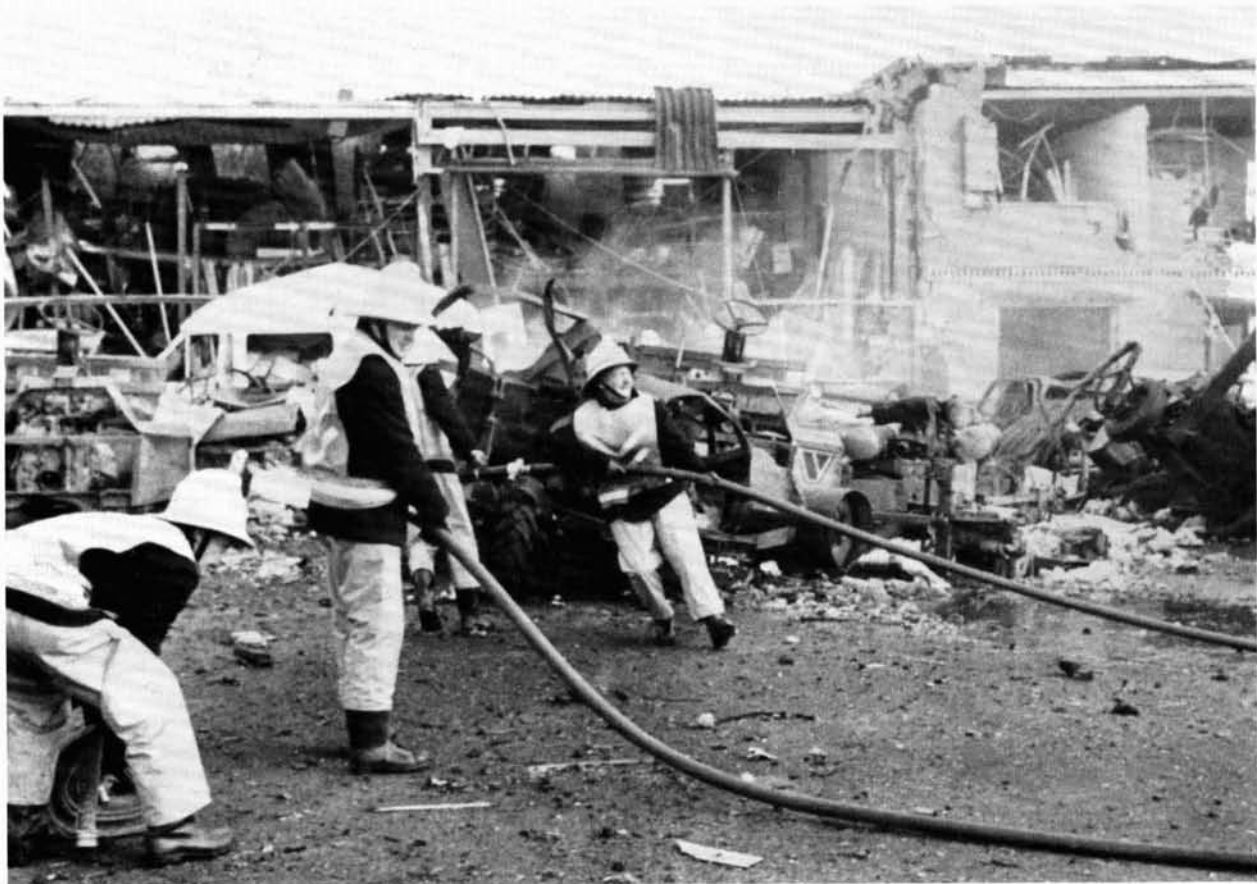
Figure 10 Blast damage to City Electrical Factors building (Photograph reproduced by kind permission of Peterborough Evening Telegraph)
