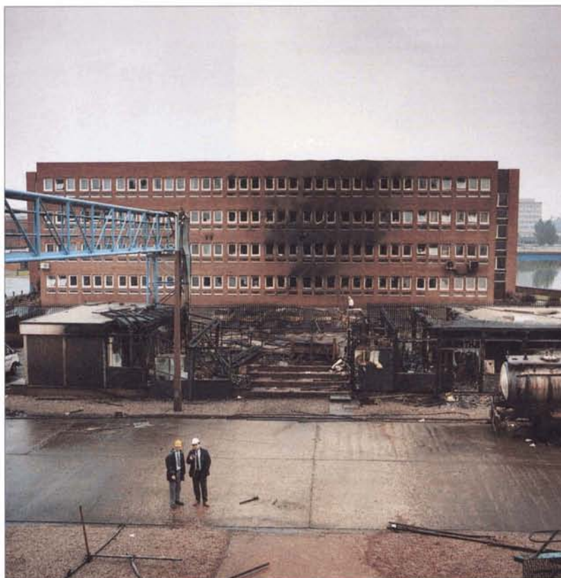
Figure 9 Photograph of roadway and buildings showing direction of the flame and scorch marks on roadway and main office block
