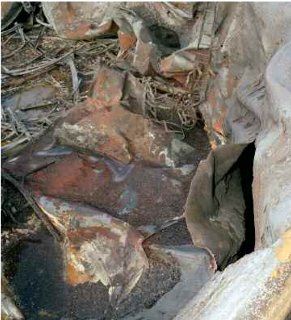
Figure 9 View into Tank 912
