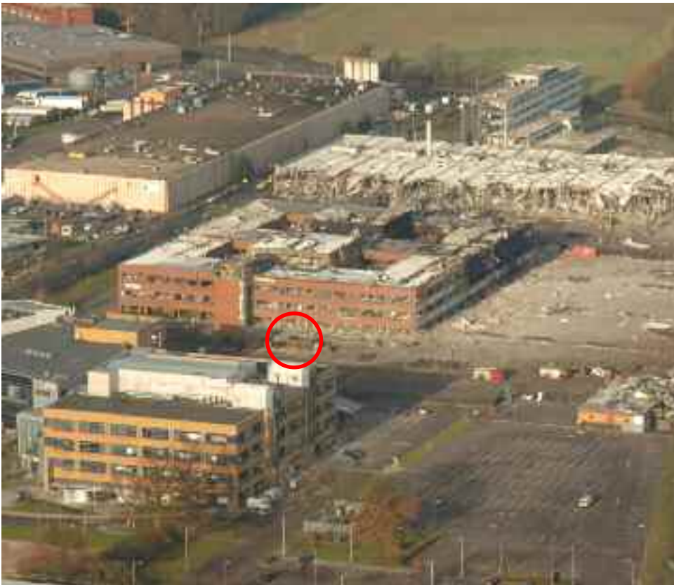
Figure 12 View looking north towards the Northgate and Fuji buildings, with the Buncefield depot just off picture on the right. The emergency generator cabin is highlighted
