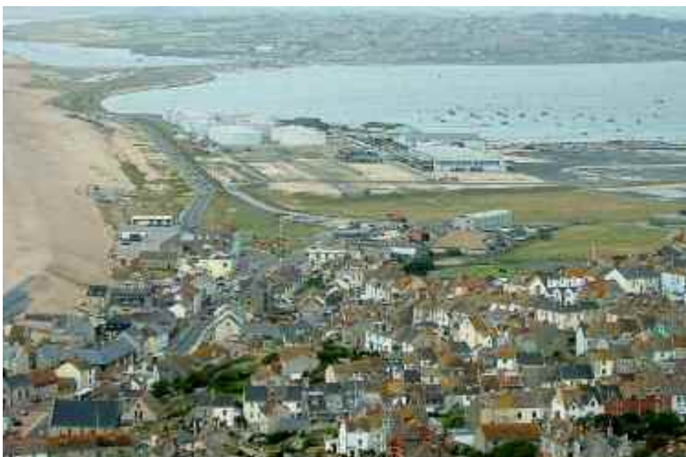
Figure 4 A view across the ex-Royal Naval Air Station and the oil storage tanks – Portland, Dorset, Southern England. The end of Chesil Beach can be seen on the left of the picture. Weymouth is across the bay joined by a road bridge, shown above the tank farm
