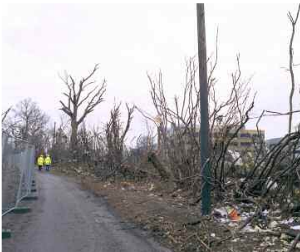
Figure 16 View south along Buncefield Lane, showing sooting of lower parts of telegraph poles and trees
