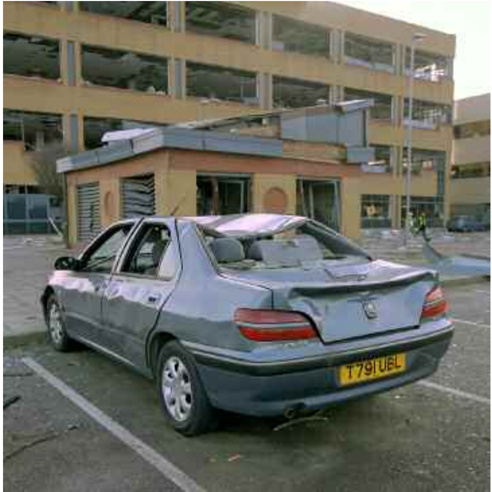
Figure 18 Damaged car in RO building car park (car facing south)
