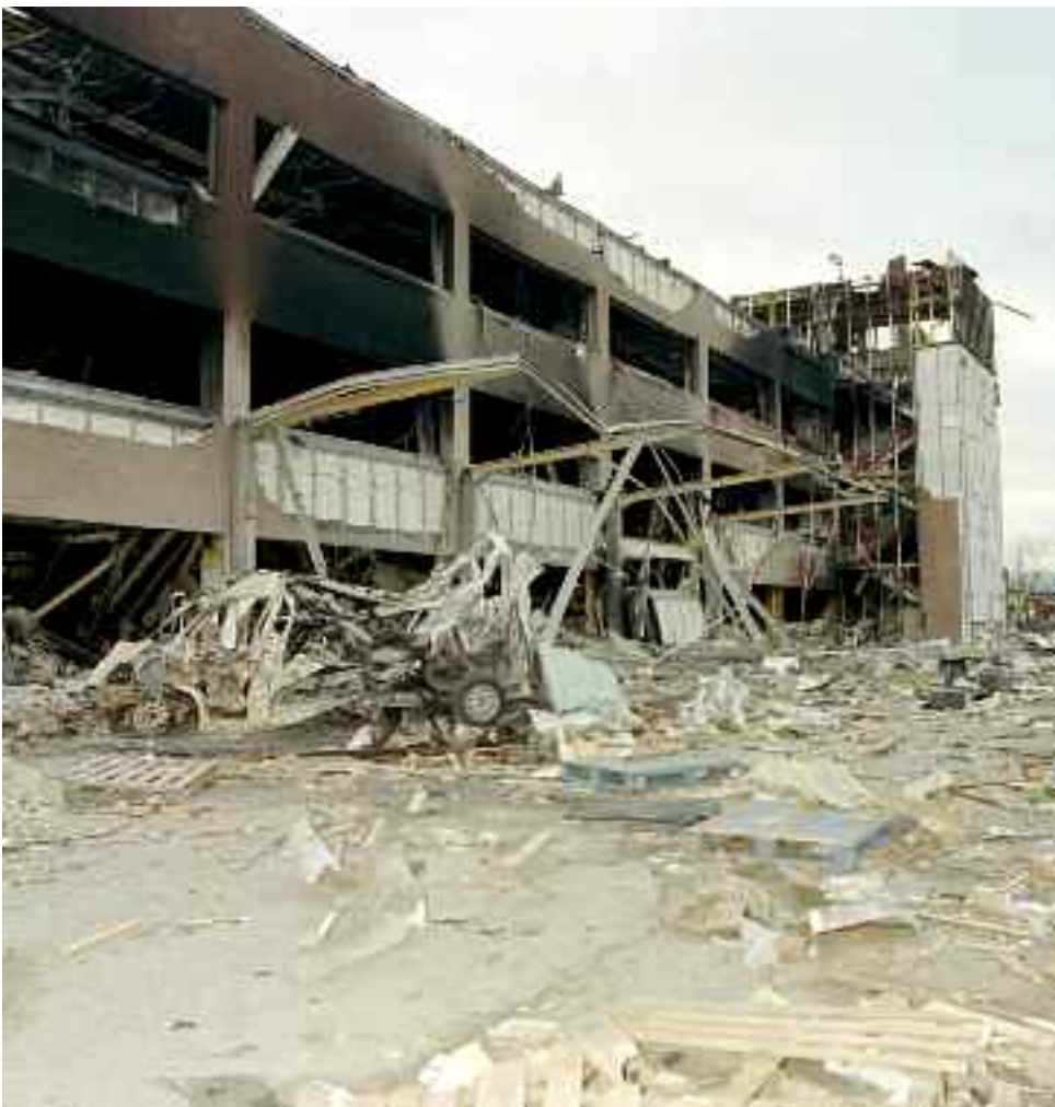
Figure 5 North side of the Northgate building
