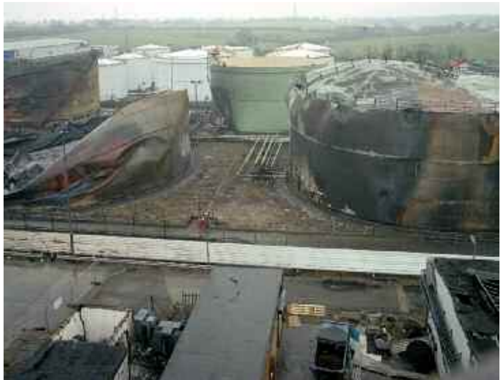
Figure 6 Looking east from the edge of the HOSL West site into the British Pipeline Agency Ltd site (Tank 4 on the left of the picture). The white tanks in the background are on the HOSL East site
