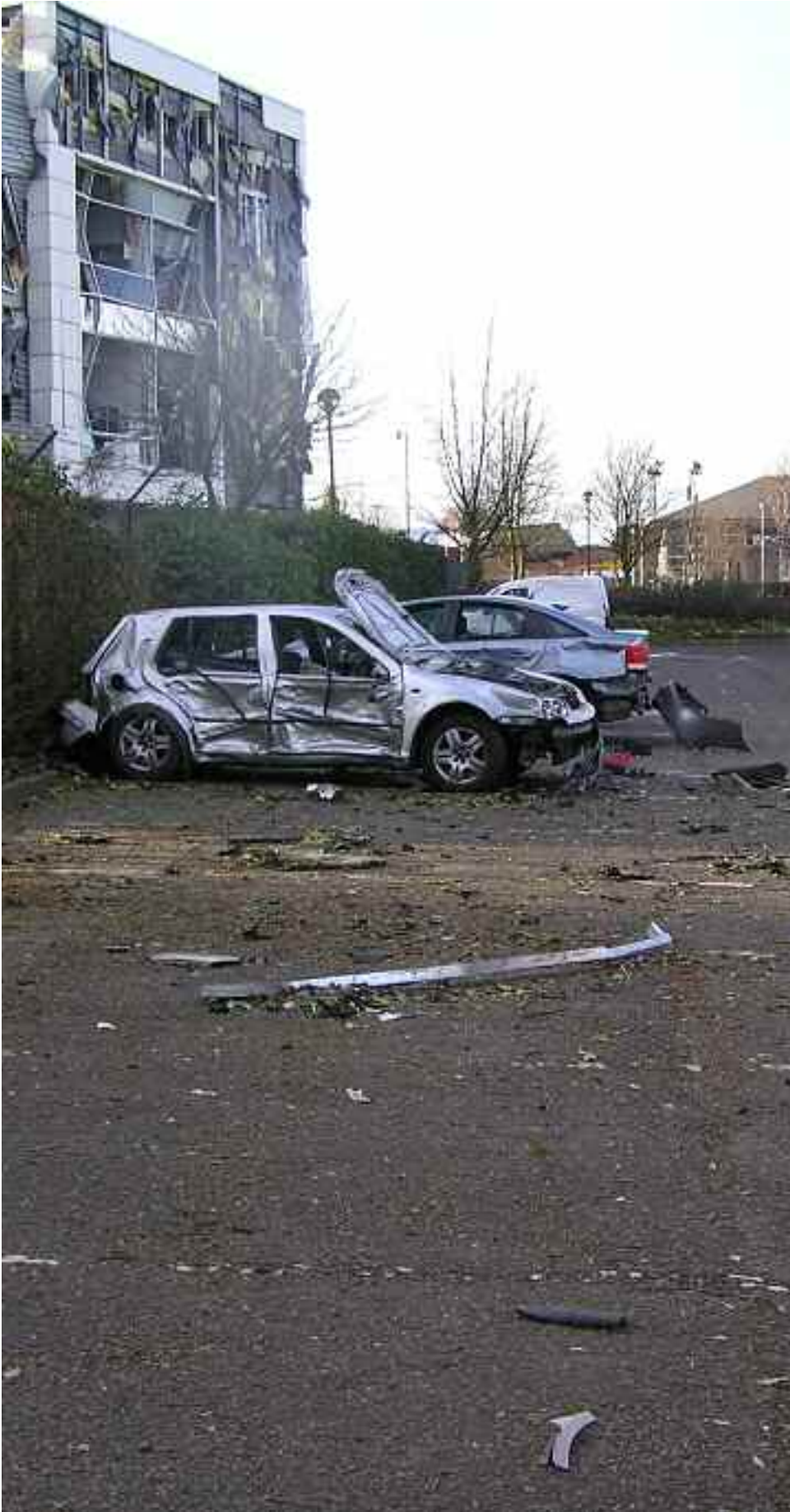
Figure 20 Damaged cars at the south-west of the Northgate building car park; Boundary Way is in the background. The picture also shows blast damage to the north-west corner of the 3-Com building
