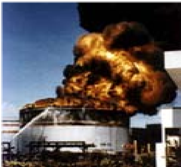
Photo E 4.1 A Tank Fire
