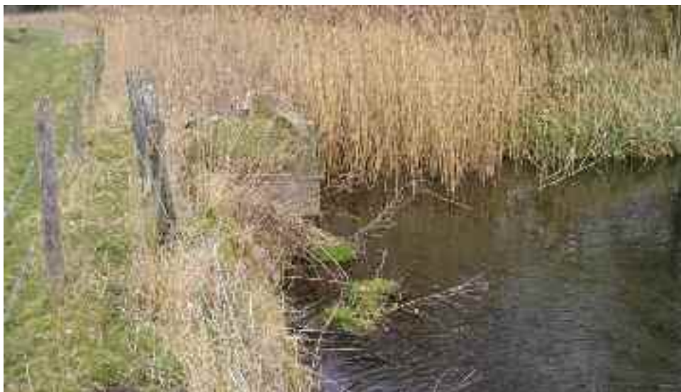
Figure 15 Picture of Maylands Tank outfall into River Ver
