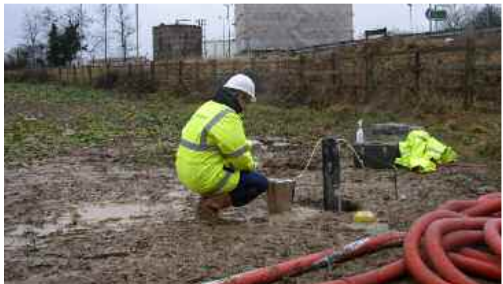
Figure 17 A new borehole at Cherry Tree Lane
