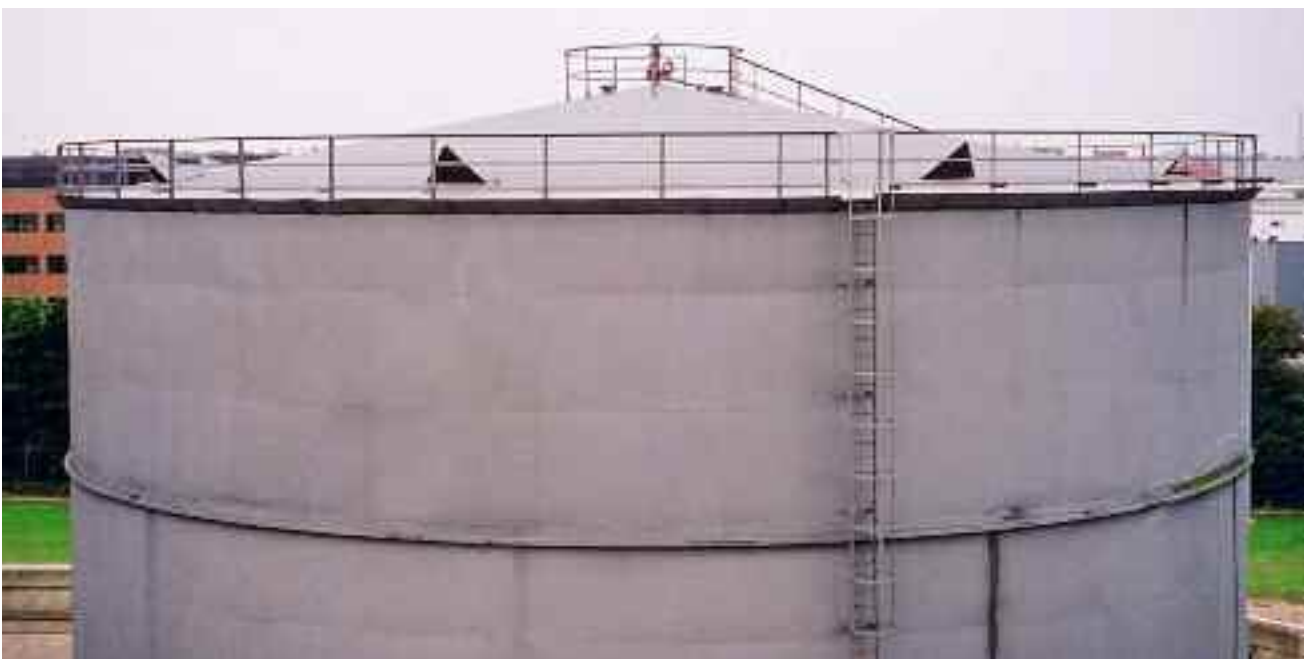
Figure 3 Tank top details before the incident
