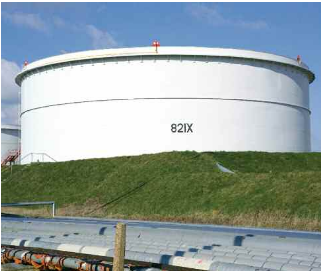
Figure 8 View of fuel tank set in earth bund
