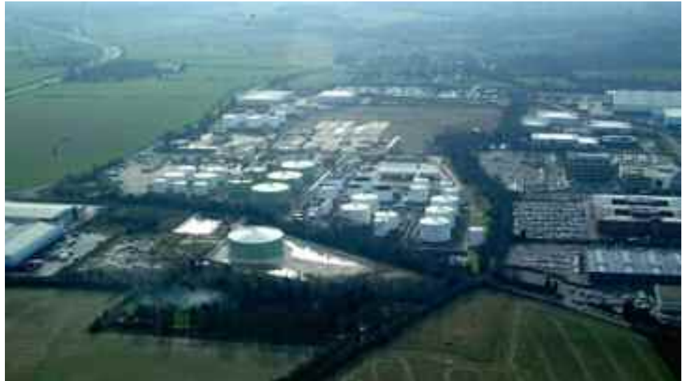
Figure 7 The area prior to incident
