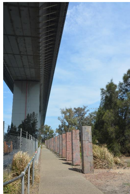
Figure 3. Memorial to workers killed at the base of the pier where the collapse occurred and 35 stone pillars representing those lost.
