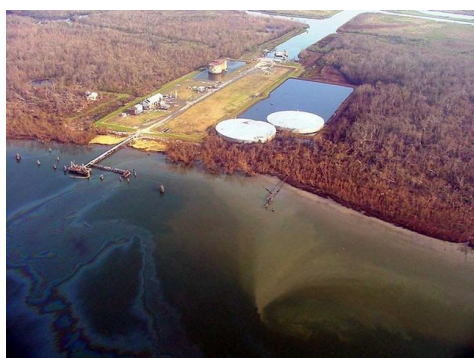
Figure 1. Tank displacement during a flood caused by Hurricane Katrina
