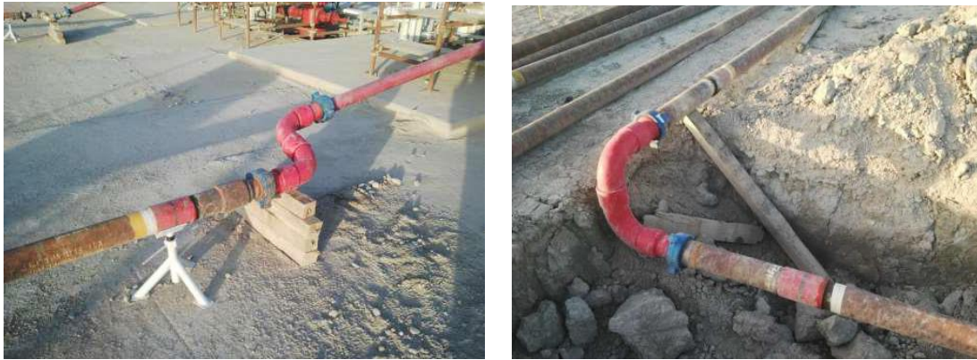
Figures 3a and 3b: Pipe supports
