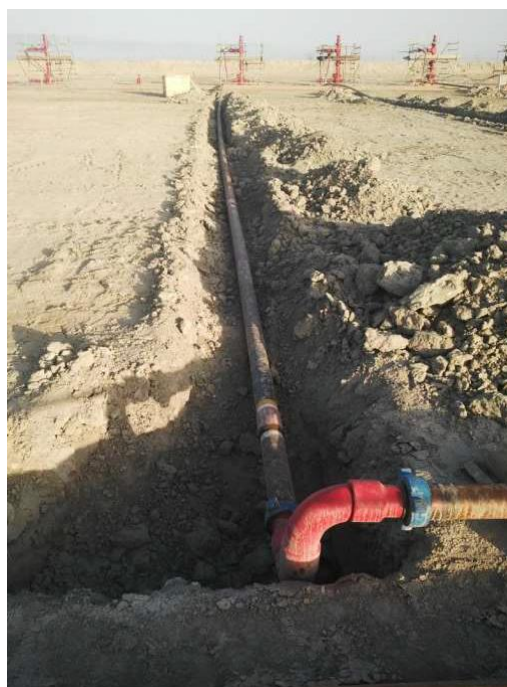
Figure 2: Flowlines leading to the main manifold.
