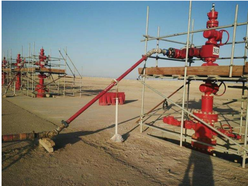
Figure 1: Operating well pad area.
