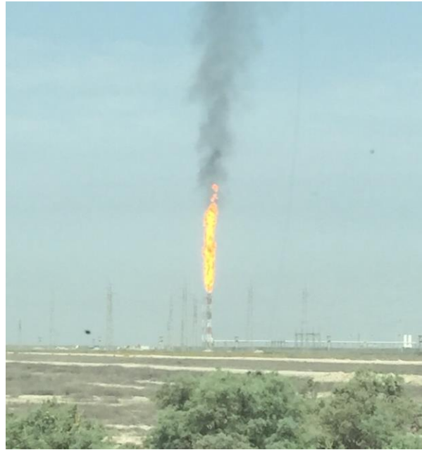
Figure 2: Continuous Flaring of Large Amounts of Gas
