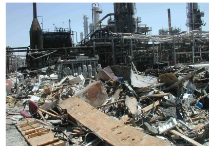
2005 Texas City Refinery Explosion (15 killed, 180 injured)
