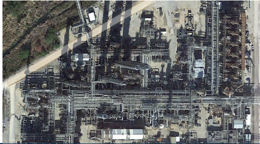
Case Study #1: Example Ethylene Unit
