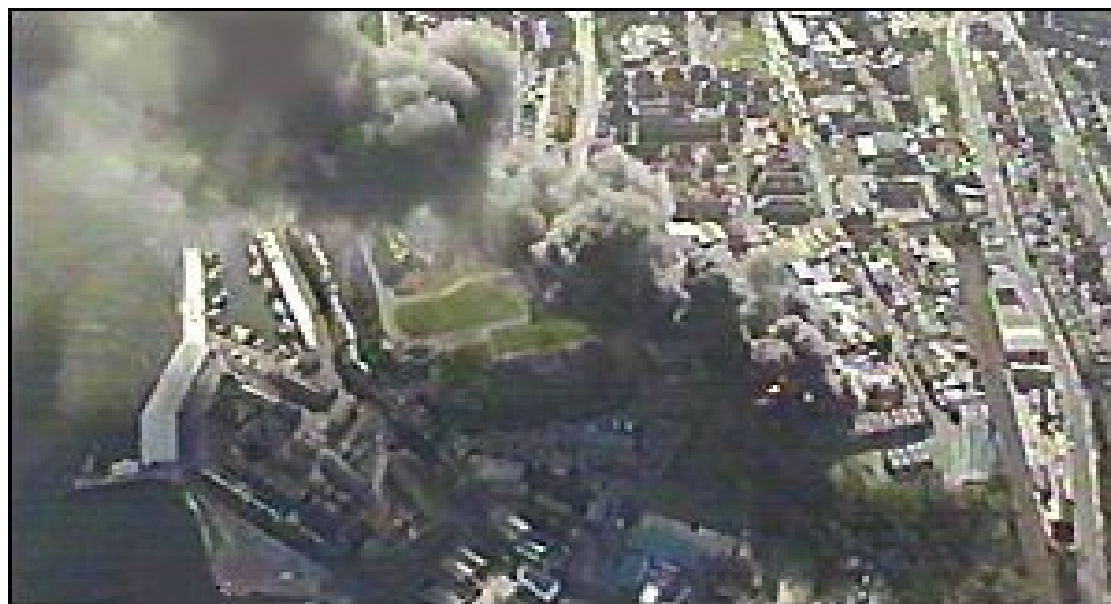
Figure 3. Distillex Ltd, fire on 12 April 2002
