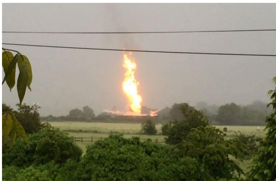
Figure 4: Fire at Oxfordshire AD Plant. Source (Nierynck, 2016)
