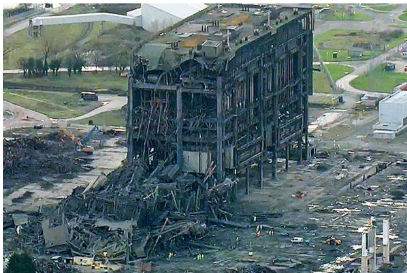
Figure 1: Didcot A Power Station Collapse. UK - 2016.
