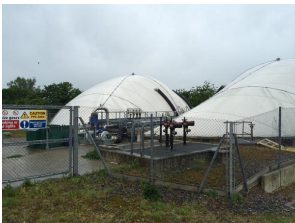
Image 5 Methane bag with braided LPS fitted.
