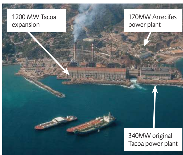
Figure 1 – The Ricardo Zuloaga Generator Complex. Tanks 8 and 9 were located at the site of the modern-day demineralised water tank (visible behind the tip of the expansion plant's middle stack)
