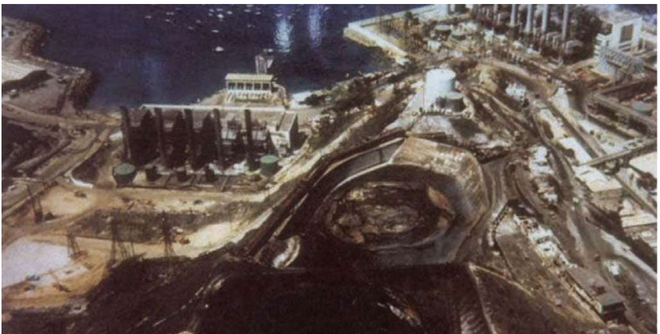
Figure 5 – Image extracted from "Incidents that Define Process Safety" shows the aftermath. Both tank 8 (foreground) and tank 9 (background) appear blackened and crumpled. Notice the steep drop-off of the dike walls and settlements underneath.
