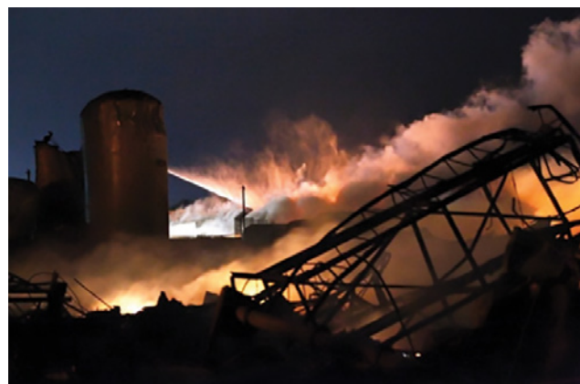
West, Texas explosion 2013
