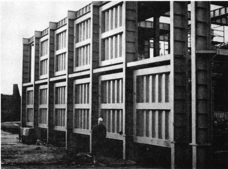
Figure 2: Completed Steelwork and Installed Wall Panels.
