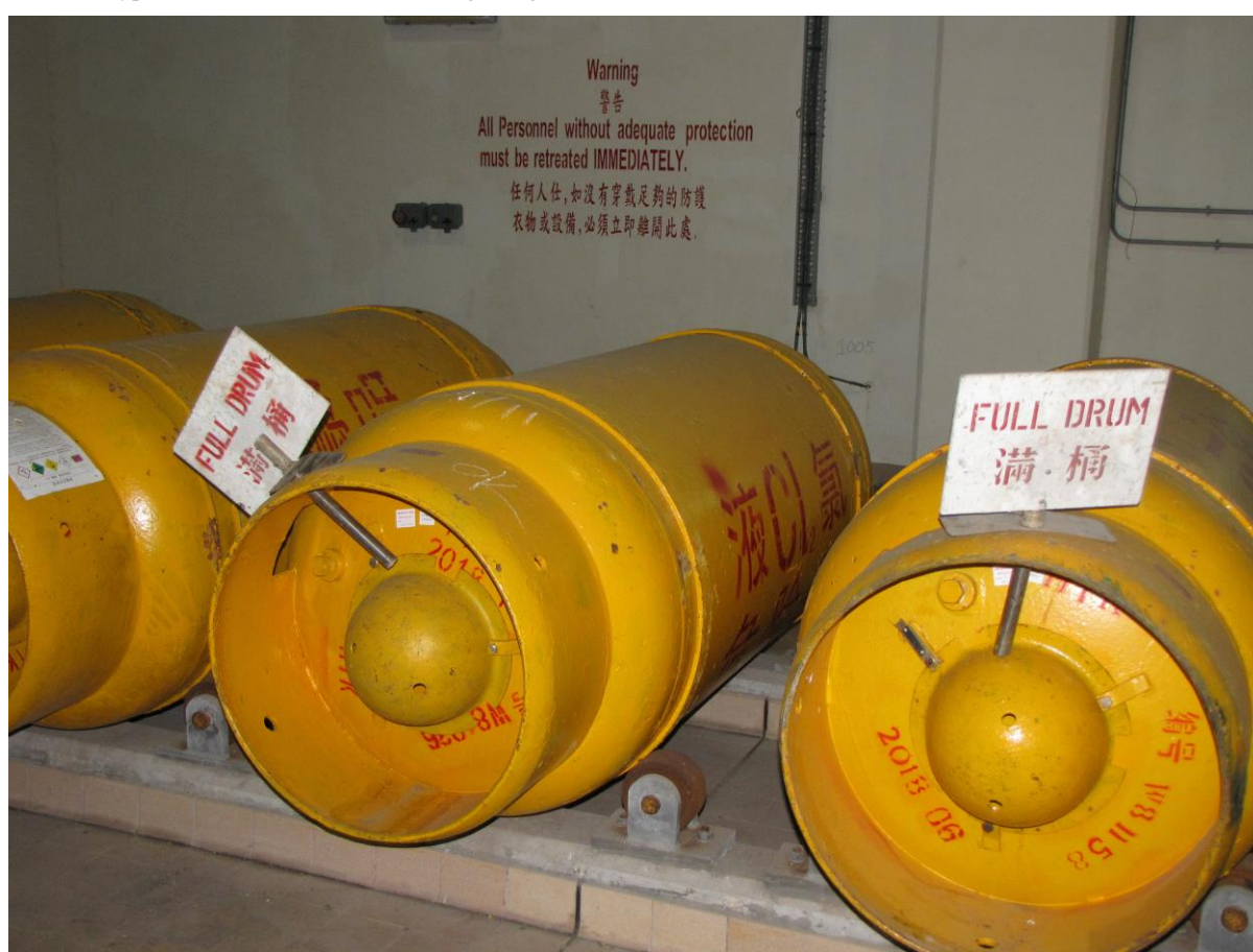
Figure 7 Typical chlorine drums used in Hong Kong (WSD, 2015)
