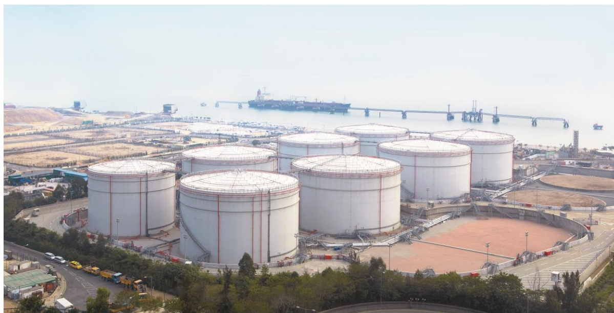
Figure 8 Hong Kong's Permanent Aviation Fuel Facility (PAFF) (photo courtesy of Hong Kong & China Gas Company Limited)
