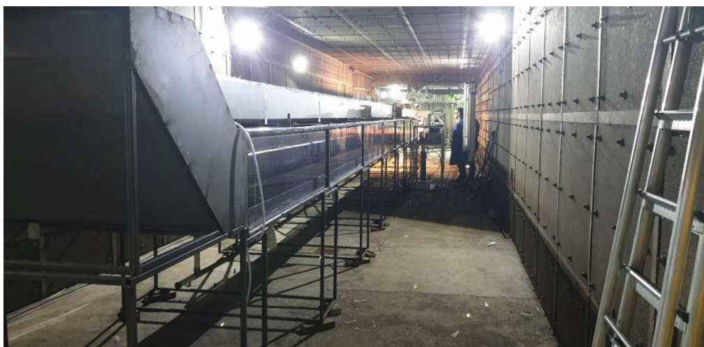
Figure 3 Scaled model tunnel as constructed.
