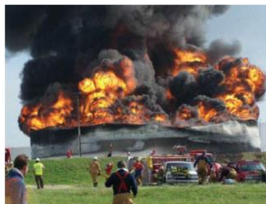
Figure 4 – Lightning-triggered fire in a gasoline storage tank (Photo credit: Assistant Chief D. Brasuell (ret.), Bixby (OK) Fire Department; Courtesy of Industrial Fire World Magazine).
