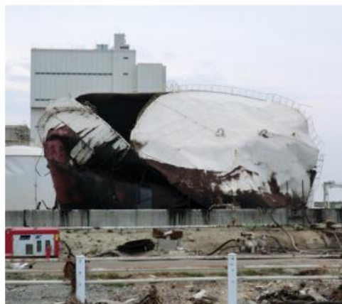
Figure 1 - Destroyed heavy oil tank at a thermal power plant battered by the mega tsunami following the Tohoku earthquake (Photo credit: A. Kouchiyama).
