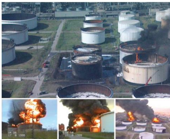
Figure 1– Fires at a refinery's storage tank farm following the 1999 Kocaeli earthquake in Turkey 5 . International response efforts were required to cope with the emergency
