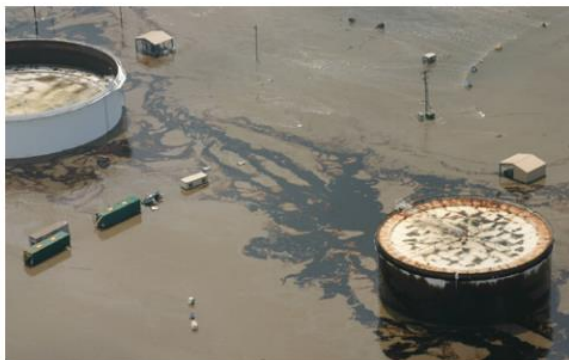
Figure 2 – Hydrocarbon release at a refinery during the Coffeyville floods in the USA in 2007. The flood exceeded the embankments protecting the town by over one metre, eventually causing a release of 400m 3 of crude oil that polluted a wide swath of land (Photo credit: Civil Air Patrol).
