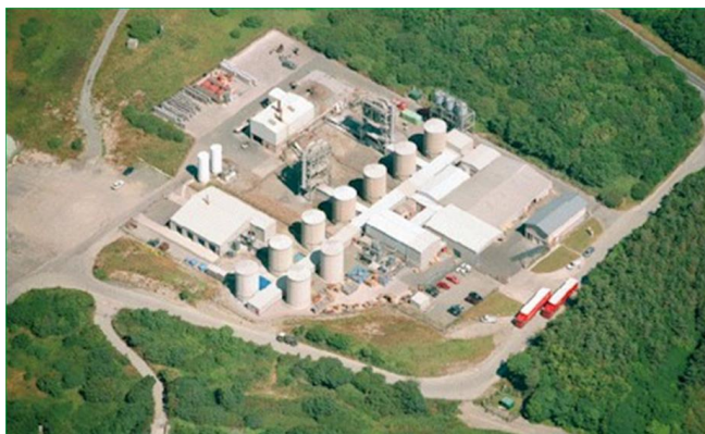
Figure 1: Aerial photograph of the site
