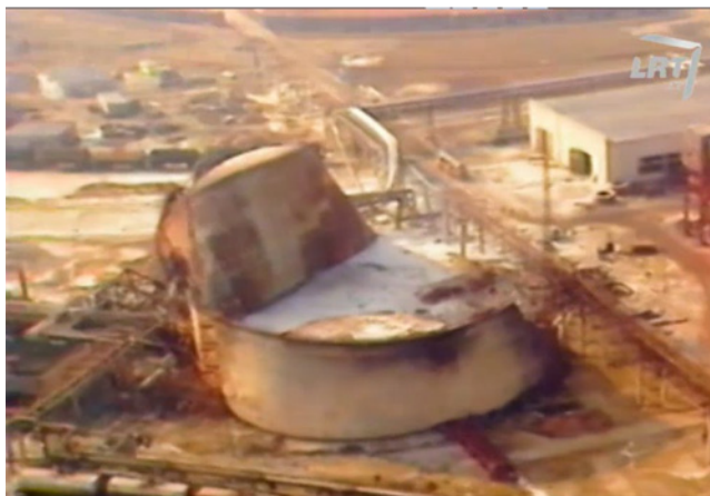
Figure 4 – Aerial views of collapsed ammonia storage tank ( https://www.lrt.lt/mediateka/irasas/2000260243/jonavos-azoto-avarija-bei-jos-pasekmes )
