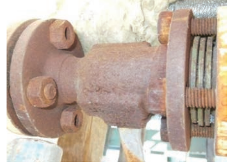
3 x spiral wound gaskets back-to-back
