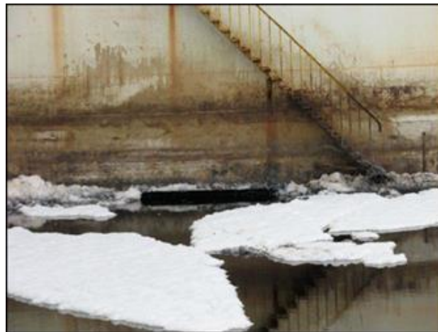
Fig. 2. Leakage following a rupture in the tank bottom
