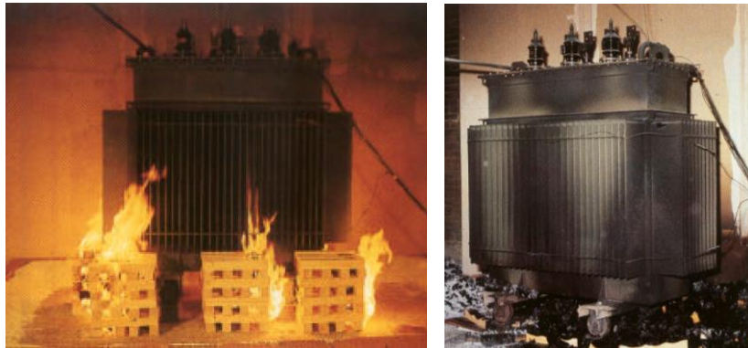
Figure 6: Transformer Victim Experiment (a) In Progress and (b) After
