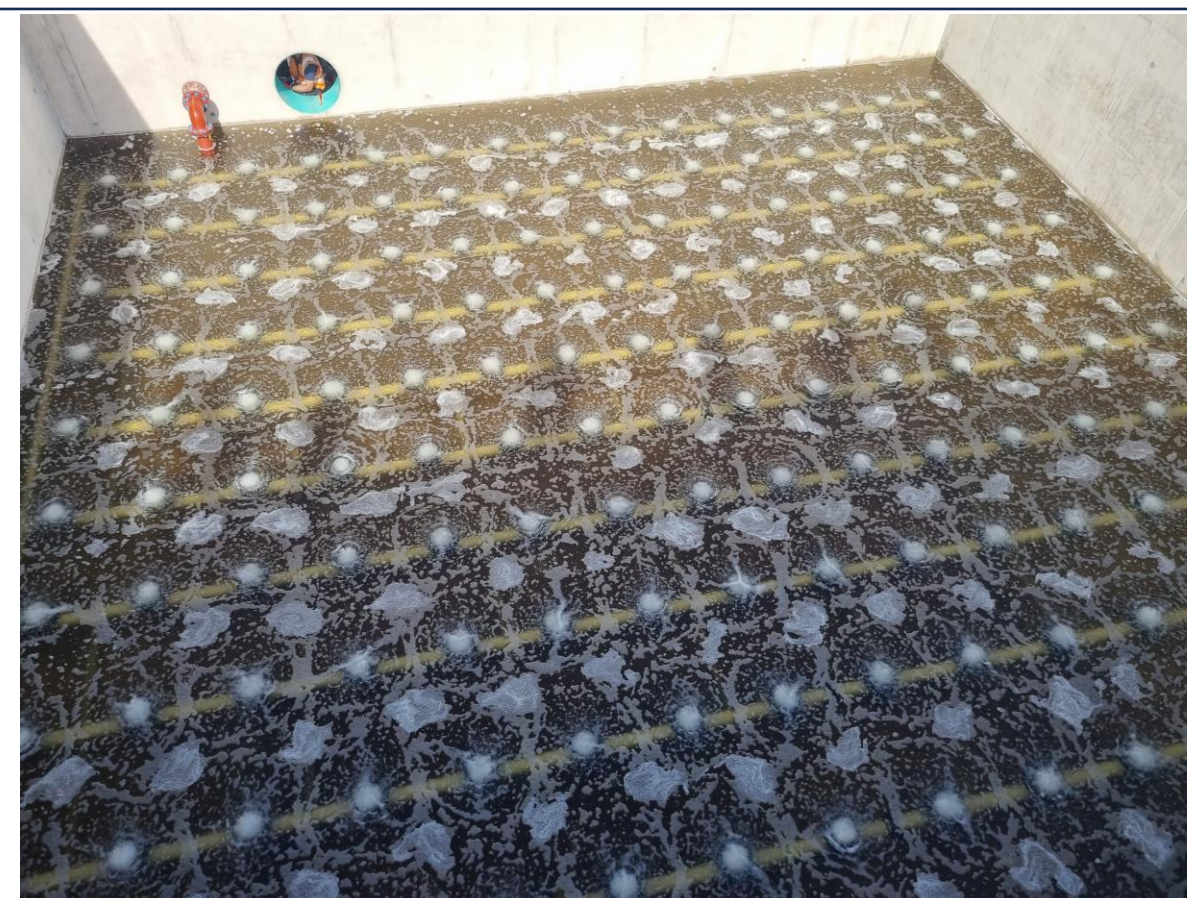
Figure 1: Wem's successful aeration pattern test in September 2024, facilitated by my programming within the commissioning process sequence.
