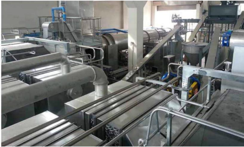
Enersavers2 - Jinhae Municipal Sludge Dryers, South Korea 2013
