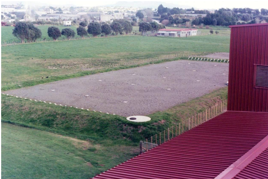
NPDC Sludge Dryer Biofilter 2000
