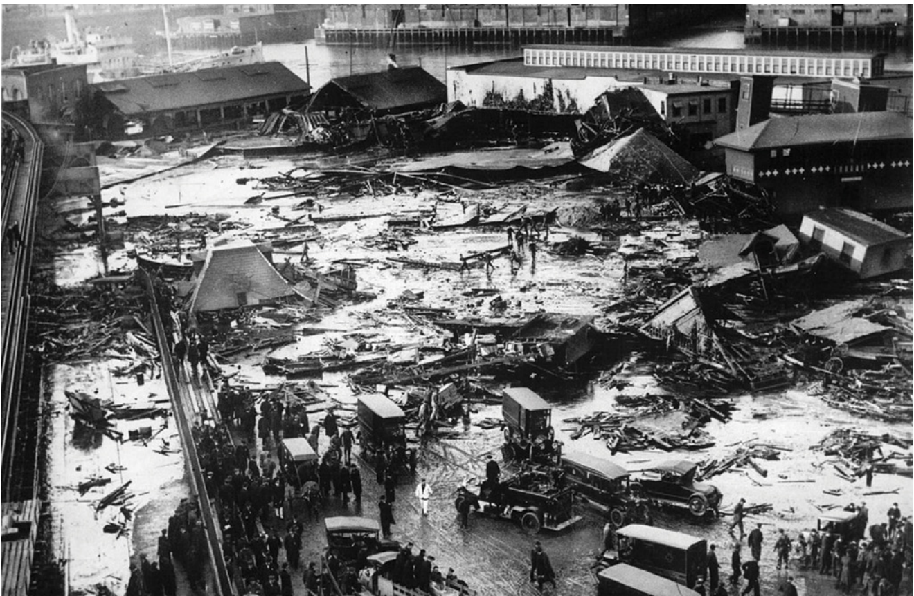
Figure 1 – The devastating aftermath of the Boston Molasses Release: Wreckage of the collapsed tank in the Background, Right, in front of the white building
