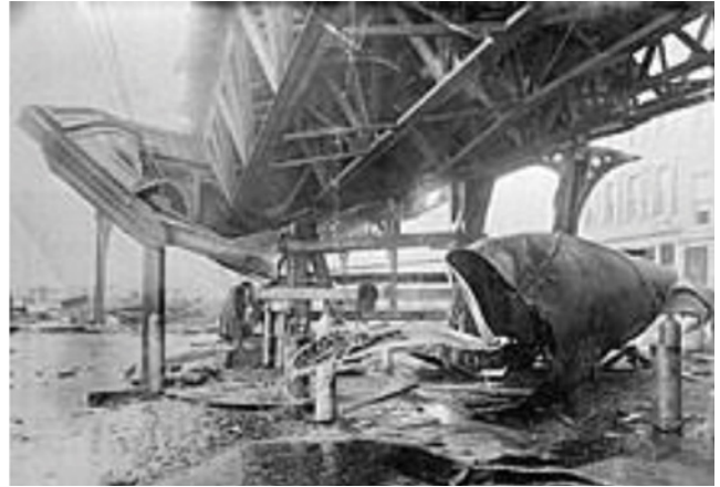
Figure 2 – Damage to an overhead railway
