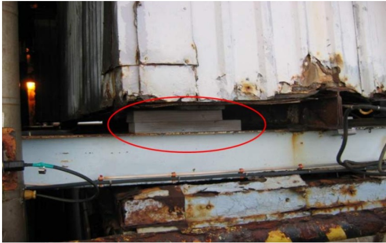
Figure 1: A temporary refuge supported on blocks when its structural integrity had been diminished by corrosion.
